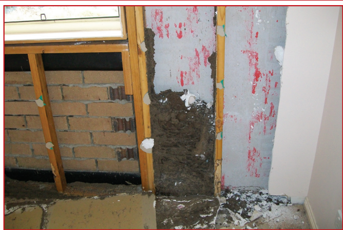
A termite subnest in a wall cavity.
